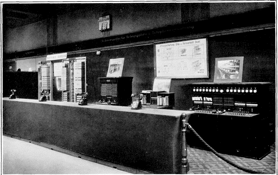
Figure 3—Model of 7-A Machine Switching Equipment at Basle, and Recording and Toll Switchboards at Safran
